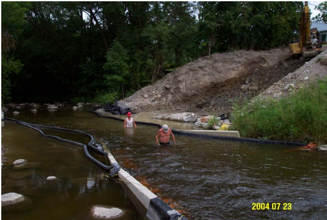
Above workers ensure that no sediment flows from the work site.
